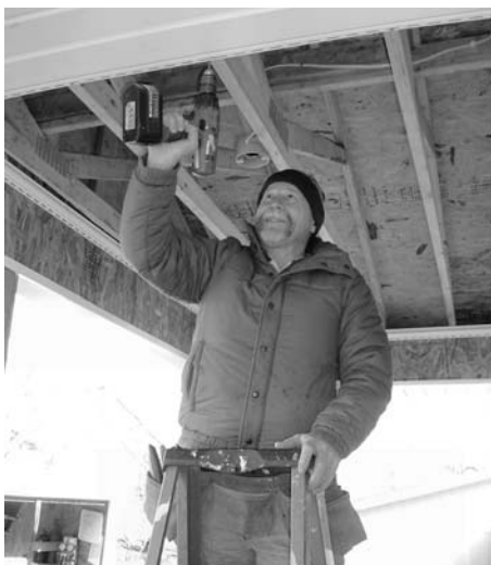
A Habitat volunteer puts finishing touches on the Jacobs porch.
