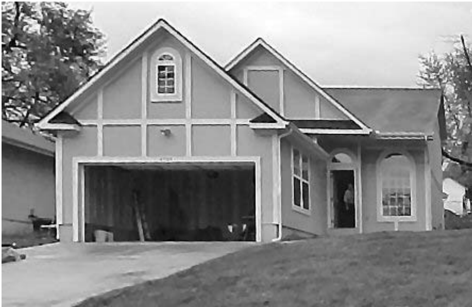
Completed infill house at 4309 N. Jackson
