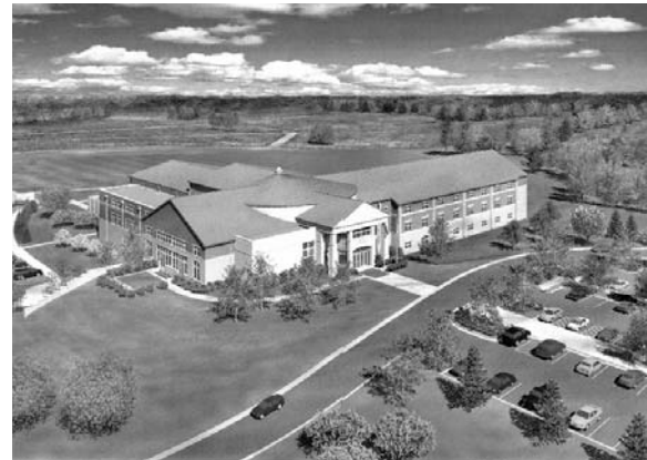
The new Police Academy will adjoin the Shoal Creek Station.
